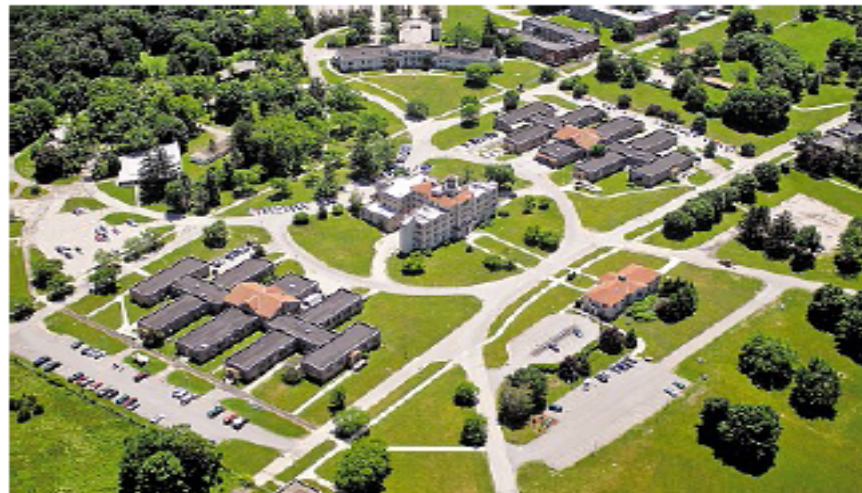
Spencer Alinsky/Poughkeepsie Journal The old hospital, which houses a dental clinic and pharmacy, appears at the center of this aerial photograph of the Wassaic campus of the Taconic Developmental Disabilities Service Organization, home to 152 developmentally disabled adults. The campus once housed 4,500. Below left , The campus power plant, which received a $7.1 million rehabilitation in 2006, among $36 million in upgrades since 2000.
